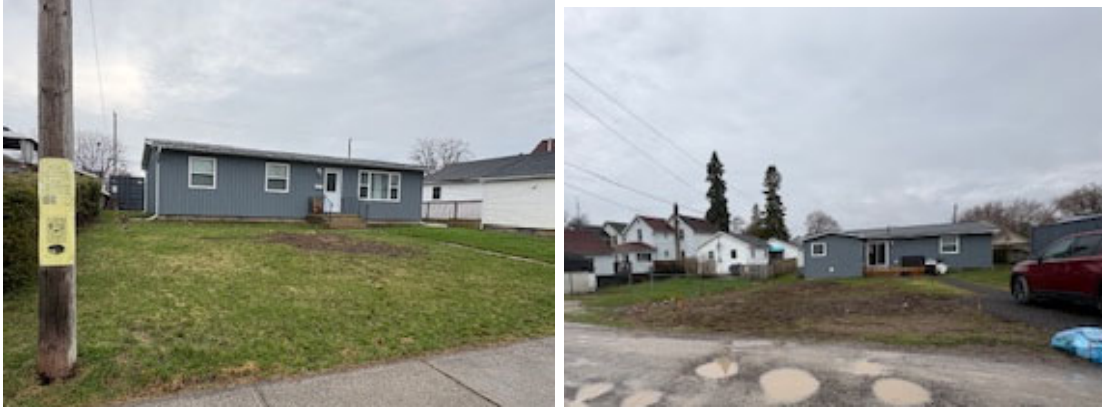
View of the front and back of the existing dwelling
